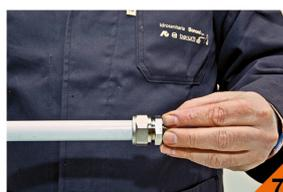
7 Pipe perfectly assembled to the connector.
