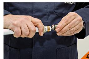
4 Insert the nut and the olive into the external pipe, make sure that the connector enter to the pipe till to touch the dielectrical washer.
