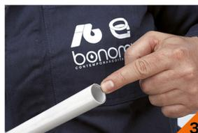
3 Verify the correct flare and eliminate the materials residues, those could damage the sealing O-Rings.
